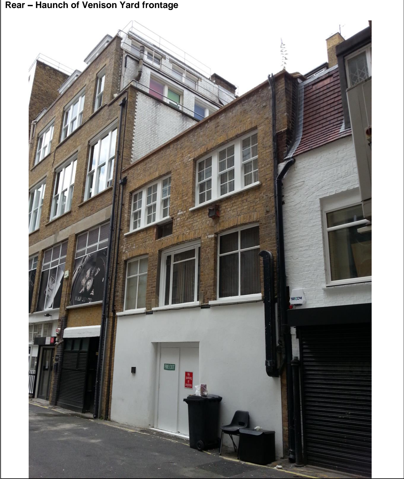
Rear – Haunch of Venison Yard frontage
